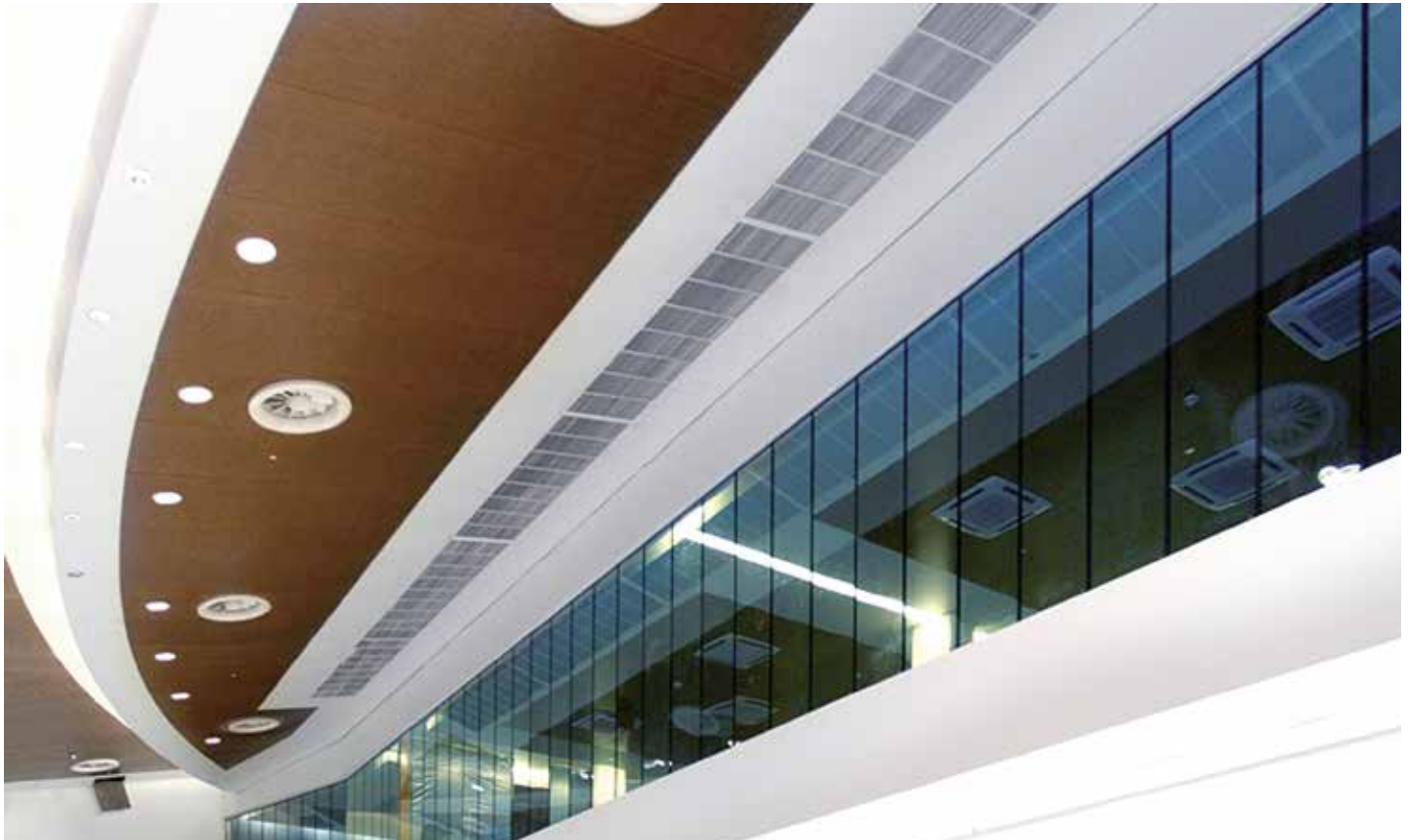
PROJECT Metro Dubai PRODUCT SYSTEMS STRUCTURE 30™
