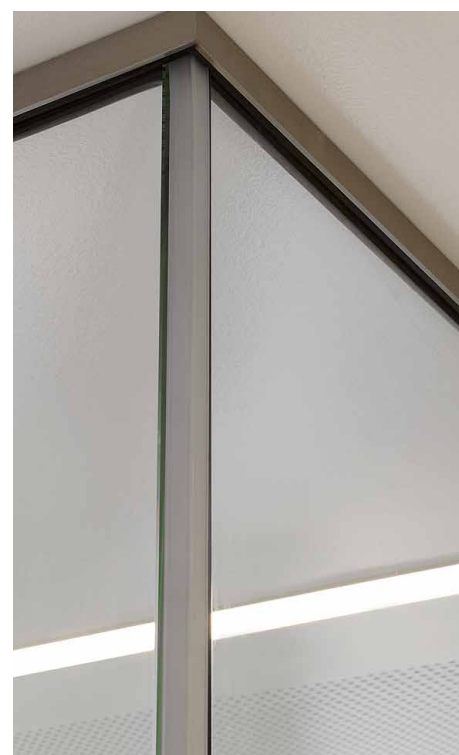
DETAIL E CLIP-IN H-profiel™
